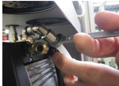
Fig. 9-13 – pull away pipe
