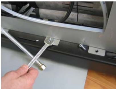
Fig. 9-12 – unscrew bolts from compressors
